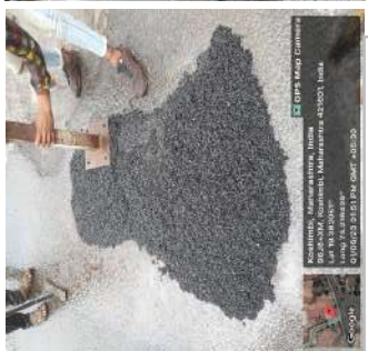
GOLDENDROP: COLDMIX POTHOLE PATCHMAKER APPLICATION
