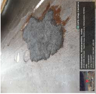
GOLDENDROP: COLDMIX POTHOLE PATCHMAKER APPLICATION
