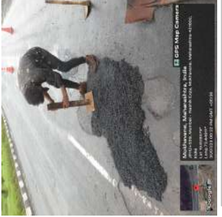
GOLDENDROP: COLDMIX POTHOLE PATCHMAKER APPLICATION
