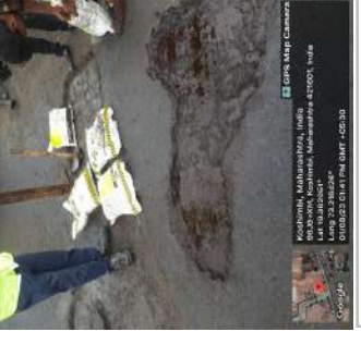
GOLDENDROP: COLDMIX POTHOLE PATCHMAKER APPLICATION
